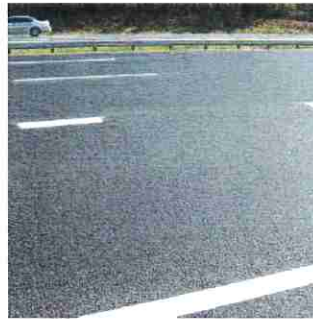
Primary streets: Asphalt
