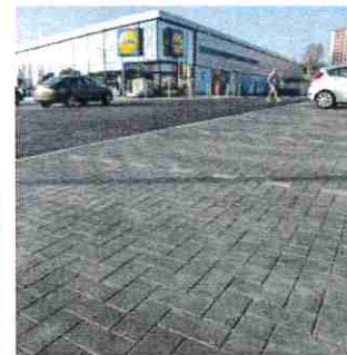
Parking bays: Block paving
