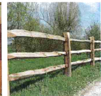
Attenuation basins: Timber post & rail
