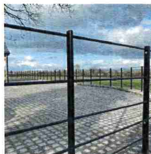
School Plaza: Estate fencing
