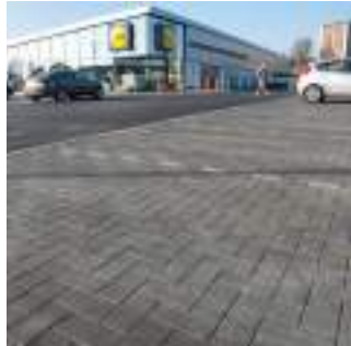
Parking bays: Block paving
