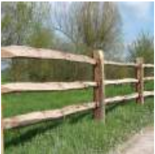
Attenuation basins: Timber post & rail
