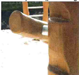
Timber Spacers (preventing toggle traps)
