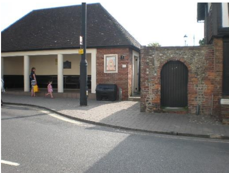
No.3 High Street, Bus Shelter
