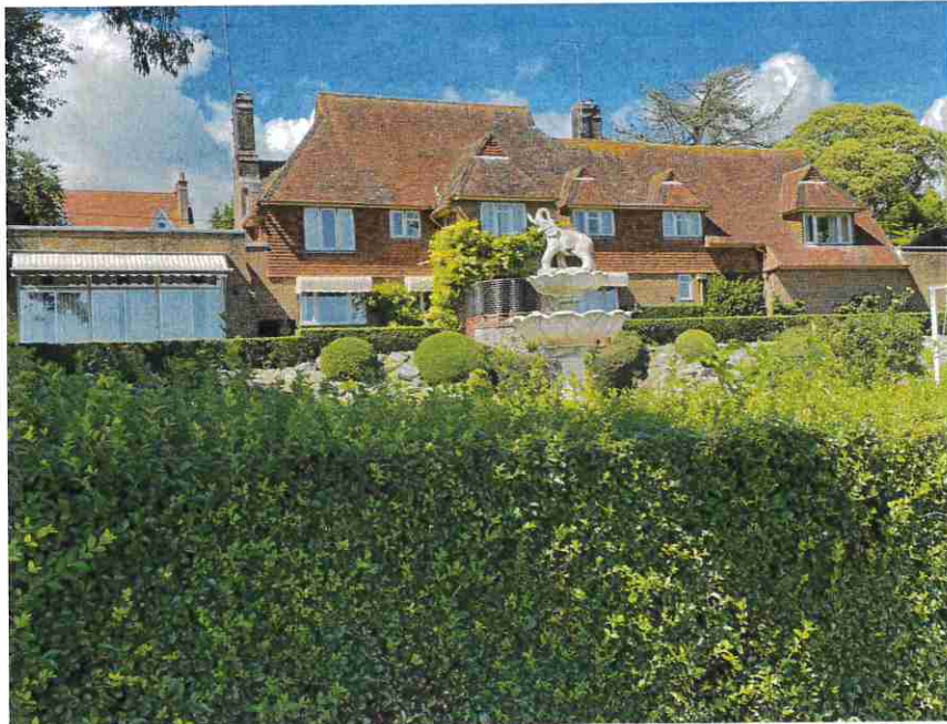
Rear elevation overlooking Clays Field
