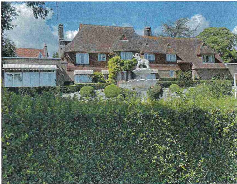
Rear elevation overlooking Clays Field
