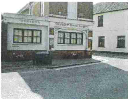
No. 1 Bramber Road, near junction with Jarvis Lane
