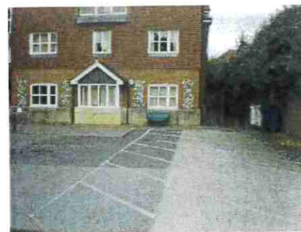
No. 6 Steyning Health Centre
