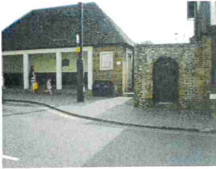
No.3 High Street, Bus Shelter
