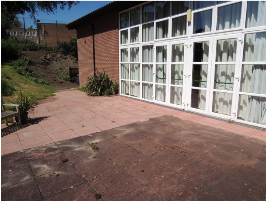
Patio at Steyning Centre
