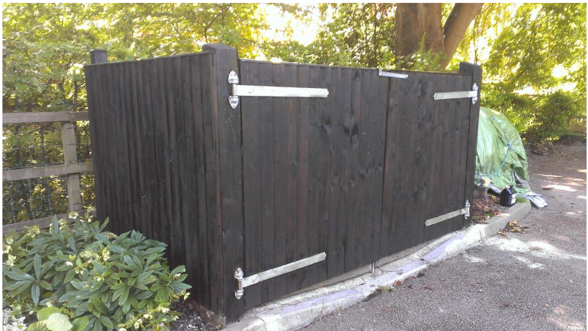
Bin Store at Steyning Centre
