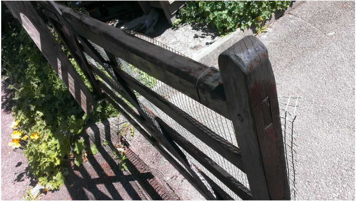
Finished gate at Steyning Centre
