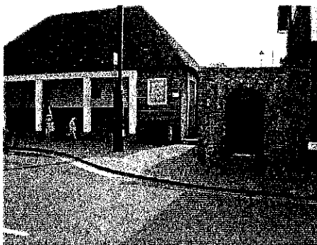
No.3 High Street, Bus Shelter
