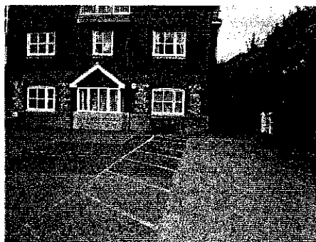
No. 6 Steyning Health Centre
