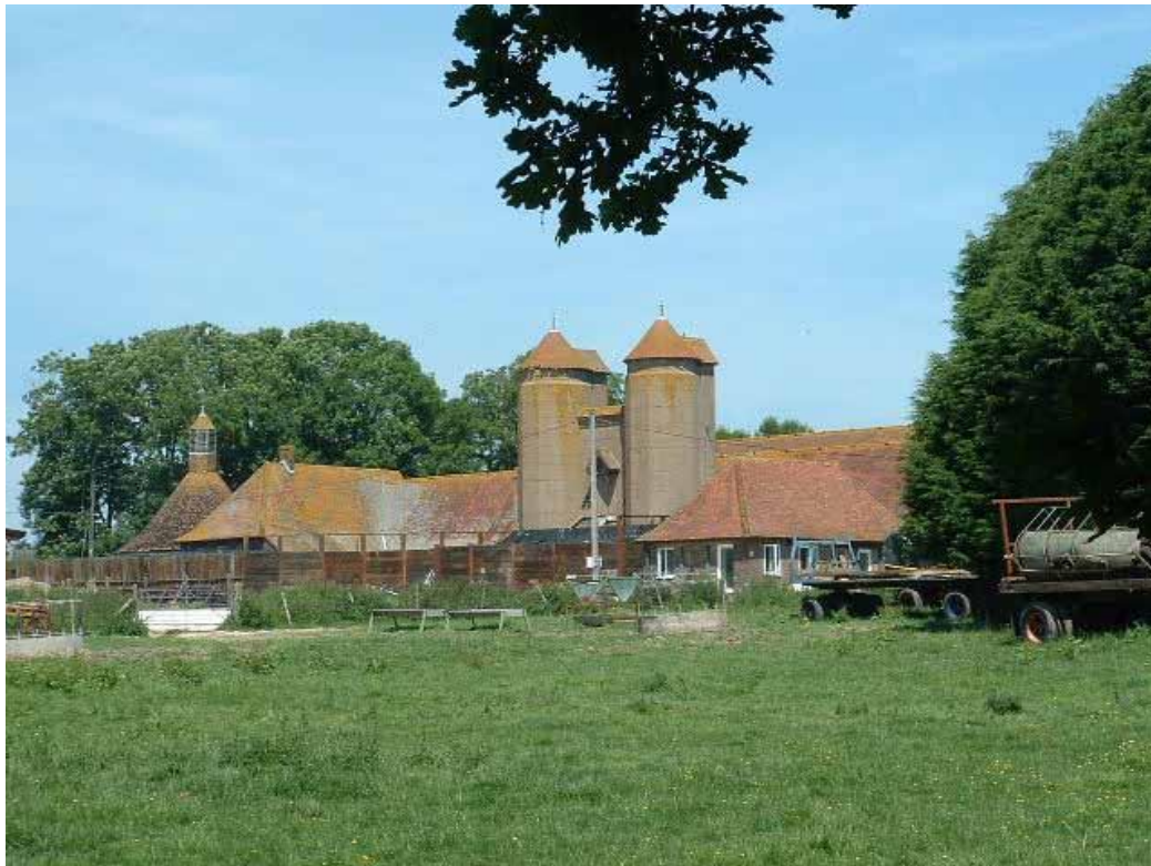
Figure 64 - Listed Wappingthorn Farm buildings
