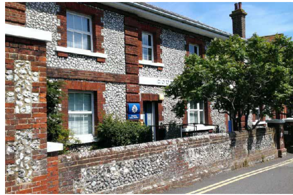
Figure 14 - Steyning Police Station
