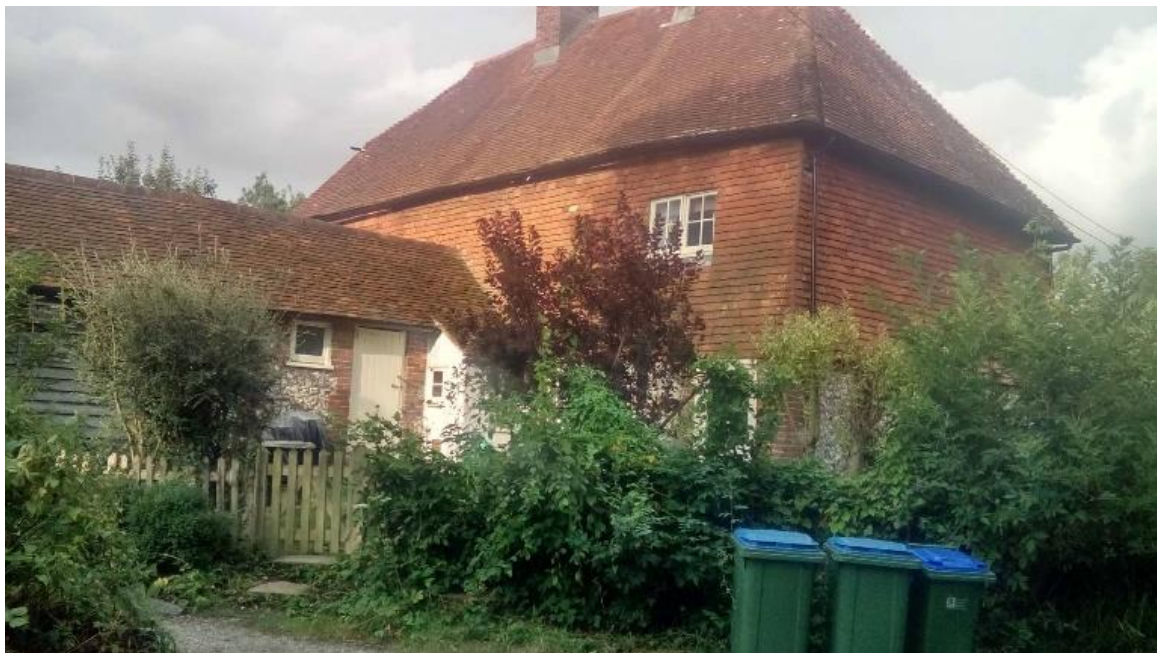
Figure 54 - Charlton Court Cottages
