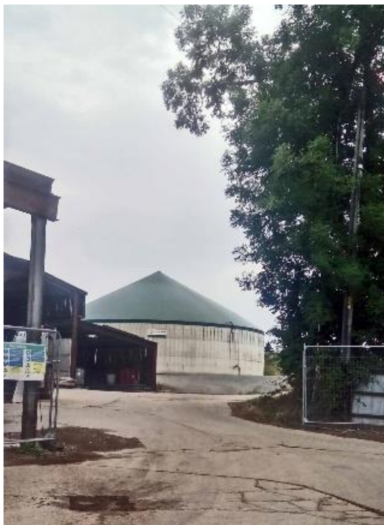
Figure 59 - Anaerobic Digester Wappingthorn Farm
