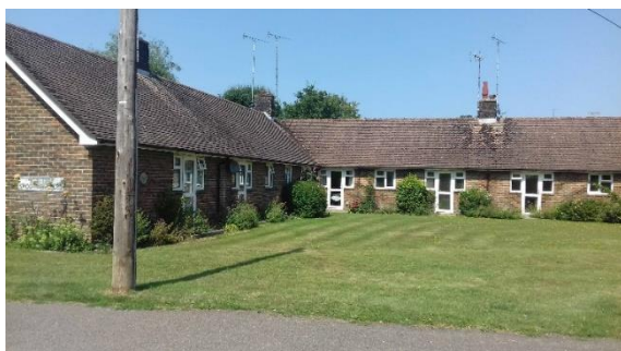
Figure 18 - Bungalows adjacent to Dingemans Court
