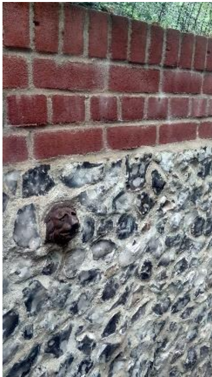
Figure 67 - New boundary wall in Mouse Lane using flint with design feature
