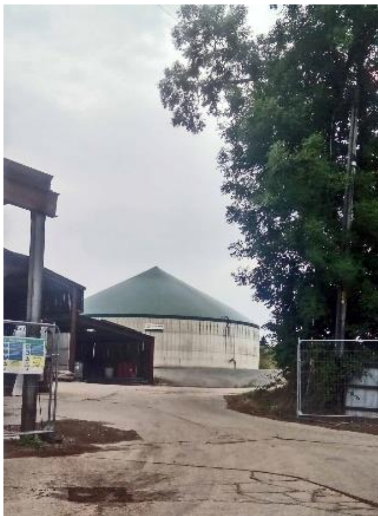
Figure 59 - Anaerobic Digester Wappingthorn Farm
