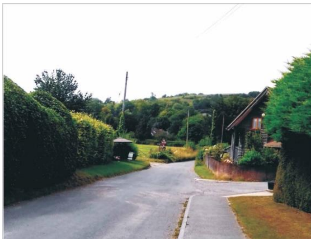
Figure 51 - Newham Lane, looking west up single track road to South Downs
