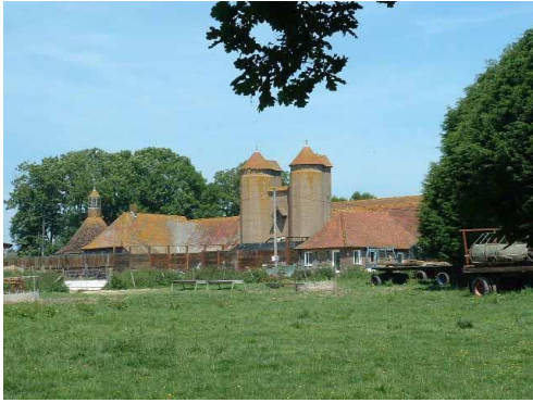
Figure 64 - Listed Wappingthorn Farm buildings
