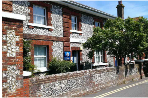
Figure 14 - Steyning Police Station
