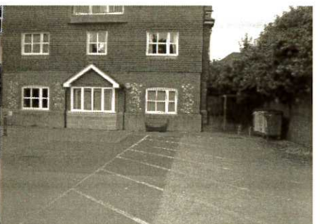
No. 6 Steyning Health Centre
