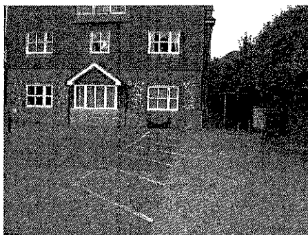
No. 6 Steyning Health Centre
