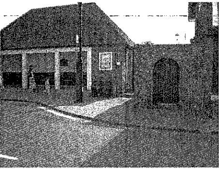
No. 3 High Street, Bus Shelter
