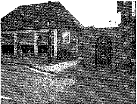
No.3 High Street, Bus Shelter
