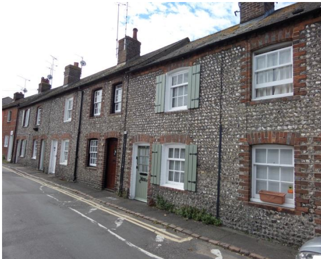
Charlton Street cottages, nos. 5-10
