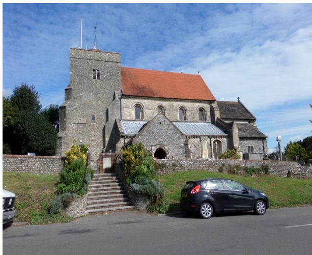
View of the Church from Church Street
